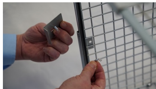
5: Fix the frame in place using the door brackets and secure with the nuts and wing bolts. 2 of the brackets without drilled holes go on the sides of the cages
